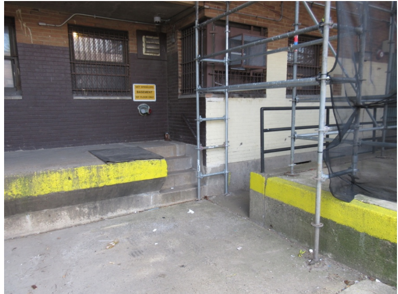
Figure 5 Loading dock and service drive
