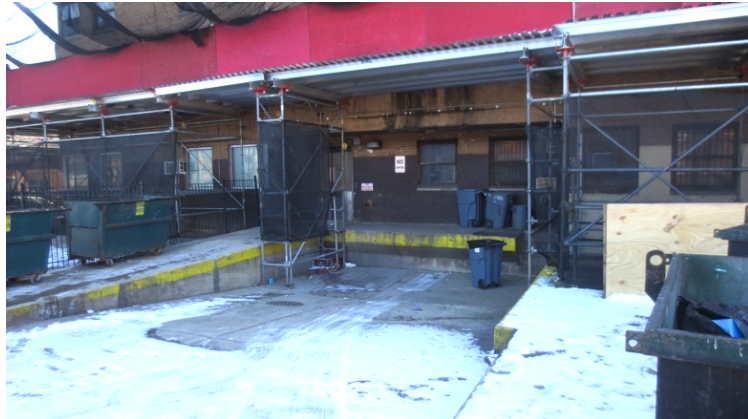
Figure 8 – Service entrance and loading dock
