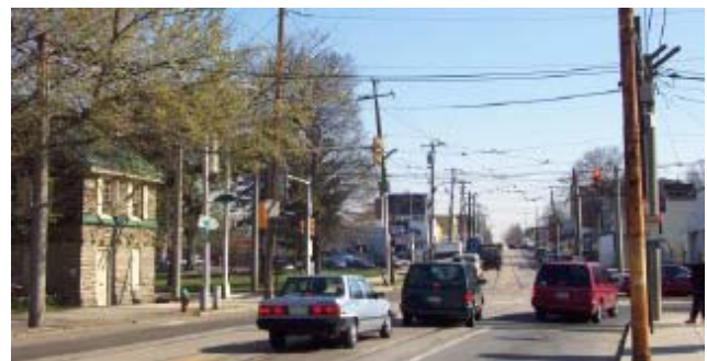
Church of St. James (above) at 68 th Street and the Blue Bell Inn (lower left) at Island Avenue are Southwest Philadelphia historic attractions. Attractive signage will welcome drivers to Southwest Philadelphia.
